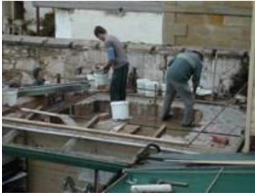
We started around the door and fire box as these parts were especially tricky. Then we worked around the side walls, gradually bringing the bricks up the slope until they met at the top where the final row of key bricks was dropped in. Sounds easy if you say it quickly, but it was fiddly and slow as each brick had to be
