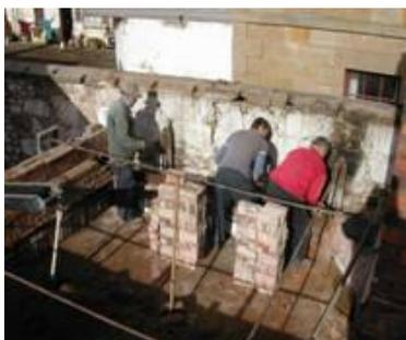
Chris collected a 3.3m piece of heavy gauge rail line and by mid-day this was manhandled into place on top of the southern oven wall to provide the support that the missing bracing strap should have supplied. Then it was a matter of tidying up the remaining brickwork, especially around the firebox.
