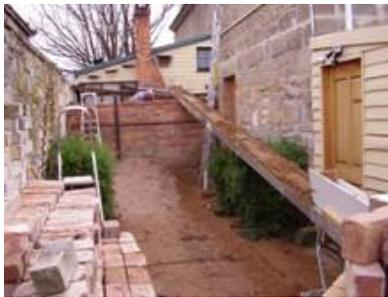
Why couldn't we apply this solution to our problem wall? We could dismantle the old bowed out wall down to oven floor level, relay the wall straight and on top of the new brickwork lay a length of railway line which would then take the roof weight and transfer it back to the perimeter steel uprights and cross rods.
