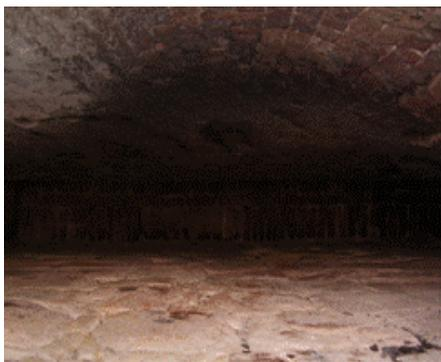
originals, laid down when the oven was built in about 1860, and they were cracking and breaking badly. We investigated quick and easy fixes such as pumping in a self-levelling concrete screed over the top of the old tiles but very soon found out that any material capable of standing up to our oven temperatures was extremely expensive; and the suppliers wouldn't guarantee the results anyway.
