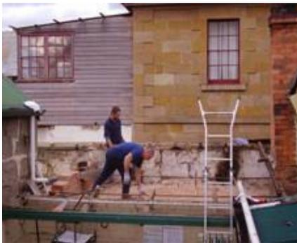
They'd already pulled off the roofing iron, shovelled off the sand and were laying into the oven crown with crowbars. We'd thought that once the first few bricks had been loosened the whole thing would crash down in a cloud of dust. Not so. Even after they'd cracked a large hole in the crown the remainder stayed up and had to be knocked down almost brick
