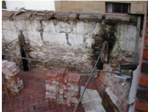
we had noticed in the area just in front of the fire box. This wall is supposed to be braced and reinforced sufficiently to take the full weight of the oven roof and the insulating sand piled on top. It's a key part of what holds up the roof dome.
