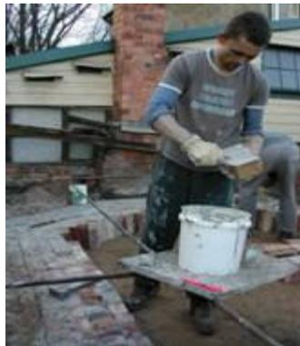
We changed our minds about the mortar a couple of times. Originally our idea was to save cost and use the premixed refractory mortar, which came in 20 kg buckets, only for the parts of the roof which get very hot; around the firebox and the centre of the crown.
