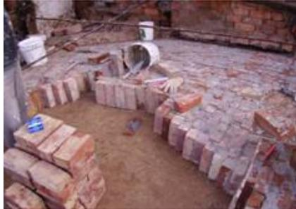
The refractory mortar was much easier to use and could be applied more thinly than standard Portland mortar; this allowed for more closely spaced bricks. We also agreed that it would be less risky in the long term to use the special mortar designed for the job, and it would be a pity to compromise the
