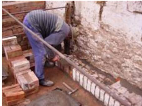
This was an unexpected setback and we could ill afford the time to demolish, reinforce and rebuild the whole southern wall from the ground up. David came up with the idea that saved us. When he had rebuilt his oven in Hobart he had laid lengths of railway line along each side for extra strength.
